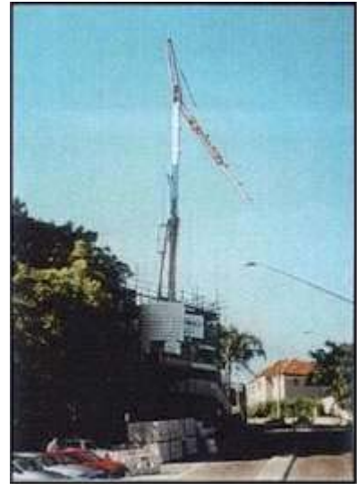
Potain self-erecting crane working from platform built on tower crane sections.
